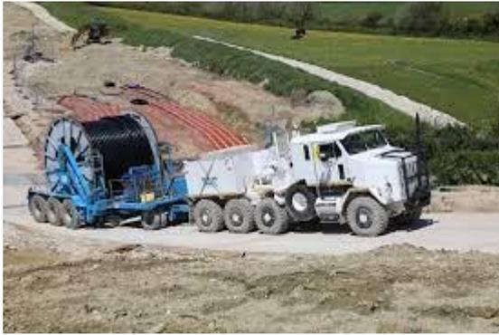
The cable comes on huge drums which weigh approximately 40 tonnes and contain about 1km of cable. Each cable is around a foot in diameter, and special equipment is used for the excavation, hauling and tunnelling (which will be used under the main roads)
